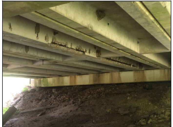
Span 2 unit 6 spalled with exposed rebar
