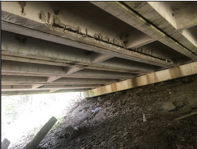
Span 2 unit 6, spall with exposed rebar.
