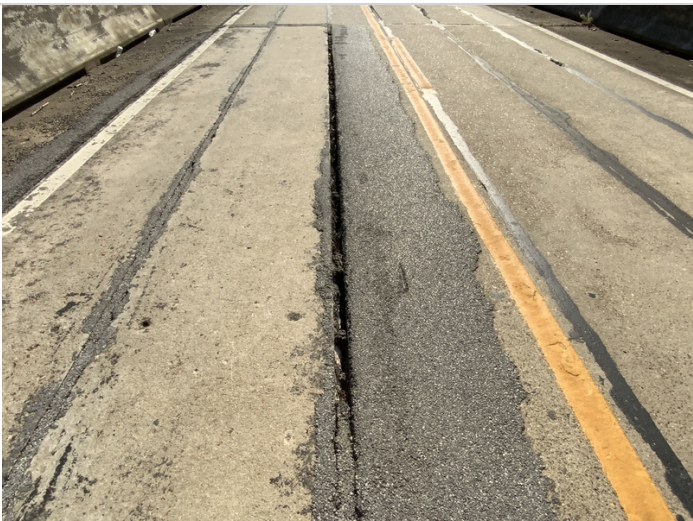
span 1, Joint between units 3 and 4 missing grout.
