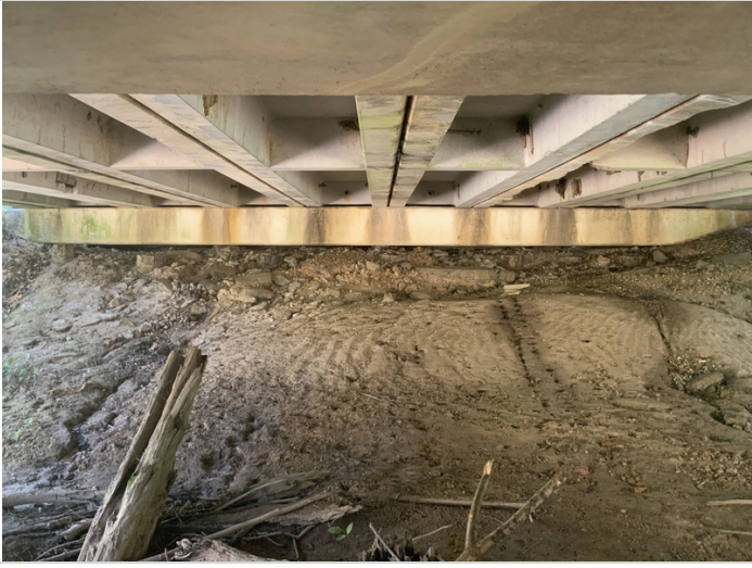
Abutment 2 (bent 3) settlement
