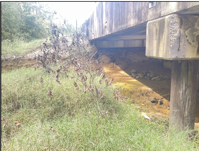
Scour under cap abutment 1
