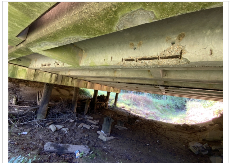
Span 1 unit 1, exposed rebar
