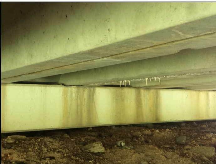
Span 1 unit 3 has numerous large spalls for entire length of the PC Unit.
