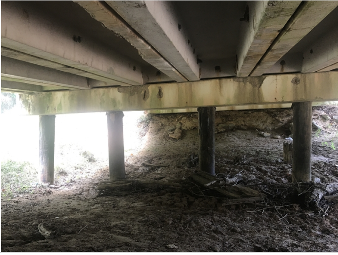
Bent 2 cap ahead face spalled delam and exposed rebar.
