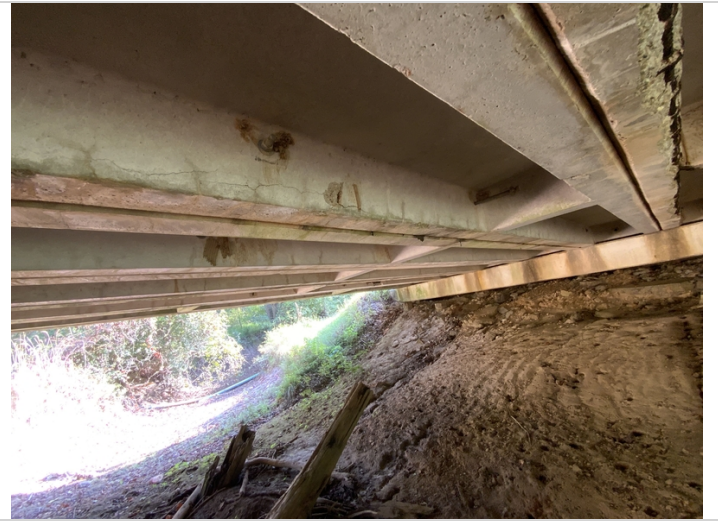
Span 2 unit 5, cracks
