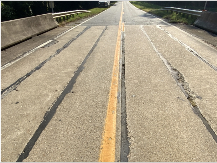
Span 2, unit 2 6 and 7, spalls
