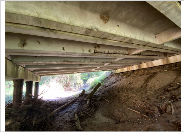
Span 2 unit 6, exposed rebar
