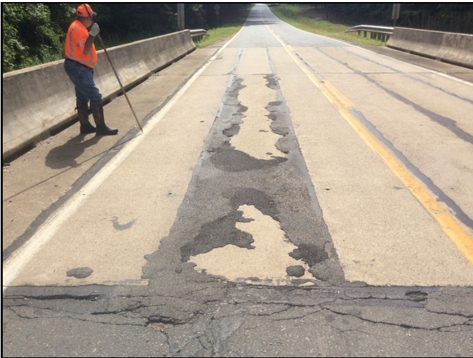
Span 1 unit 3 has numerous large spalls for entire length of the PC Unit.
