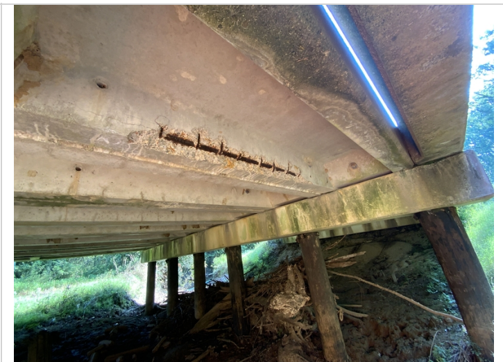
Span 1 unit 8, exposed rebar
