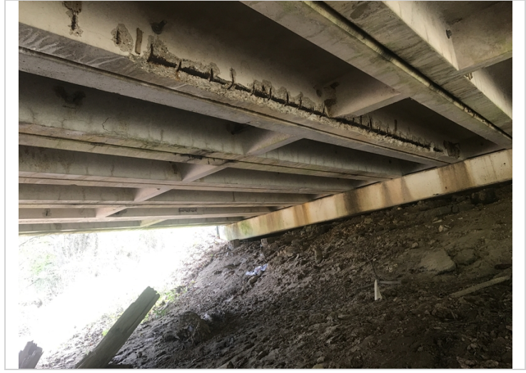
Span 2 unit 6, spall with exposed rebar.
