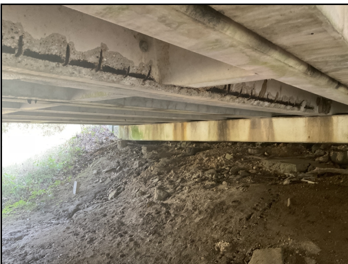
Span 2 unit 6 spalled
