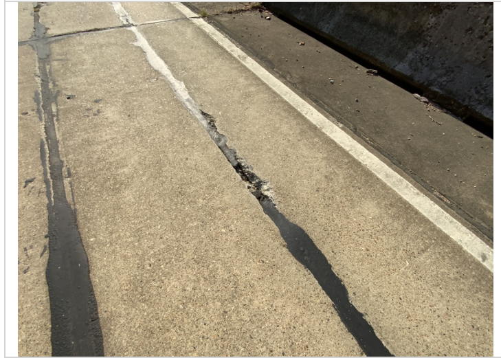
span 1, Joint between units 6 and 7, missing grout.
