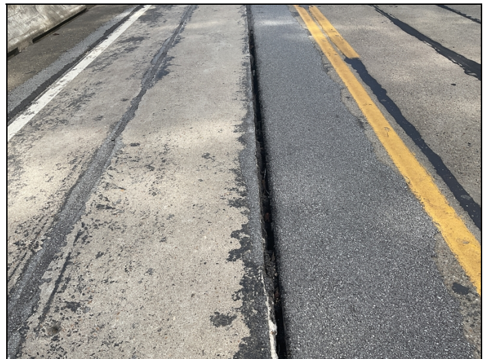
Grout missing between units 3 and 4 span 1
