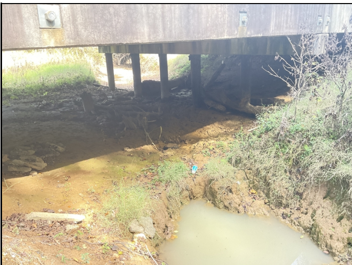
Span 1 scour Rt. side with silt and sediment built up in the stream bed
