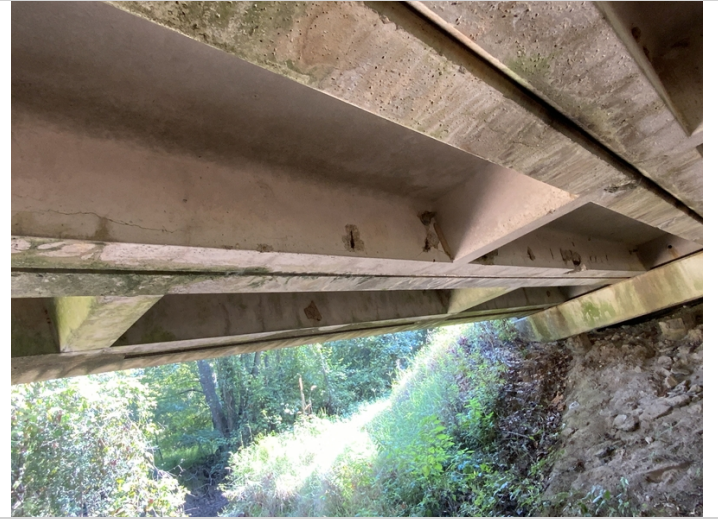
Span 2 unit 2, cracks, and exposed rebar
