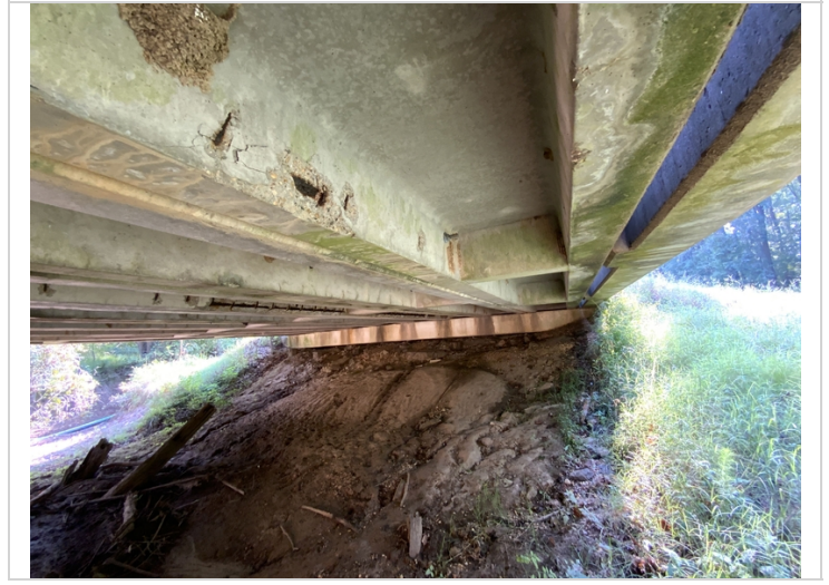
Span 2 unit 8, exposed rebar
